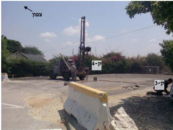
Fig. 5 Porter School - Soil Survey
